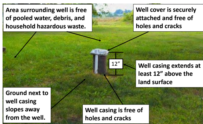
Figure 1: Photo of a properly constructed well.
