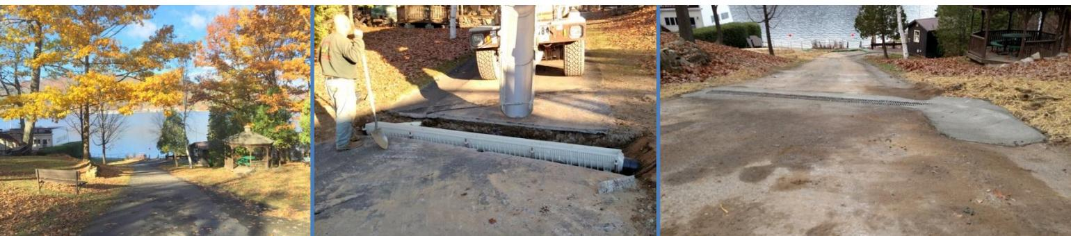
Trench drain to divert water to dry wells before (left), during (middle), and after (right).
