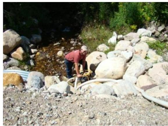
Clinton County SWCD's Dave Wilfore, District Technician, adding hydromulch (left) and pumping water (right) into the hydroseeder to seed roadside ditches.
