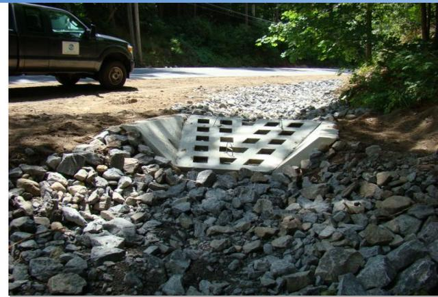
Sediment basins help to reduce the amount of sediments that enter our water sources. This one was installed in the summer of 2016 (top), and was tested out in some spring thawing February 2017 (bottom)!
